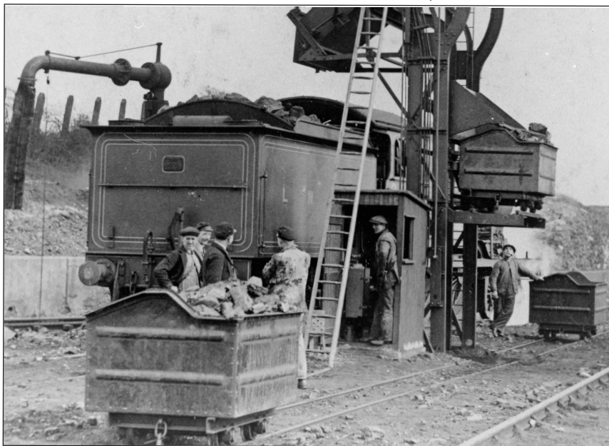
The coaling bunkers about 1950, with coal being hoisted and loaded into a locomotive with the water hose far left. The engine shed was situated further up the line towards the station
