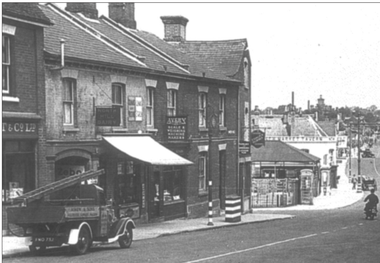
The entrance to the former Cistern Yard, behind the parked vehicle, with Avery Scales, the Coach and Horses, Cattle Market and New Market Tavern in the 1930s
