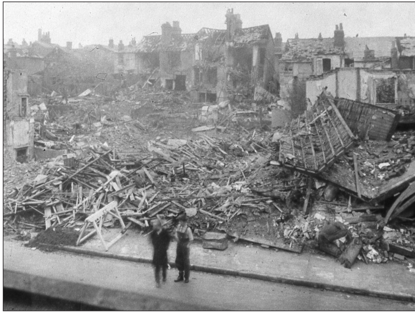
The scene of the destruction the following day caused by the bombs which fell on Chapel Street and West Street
