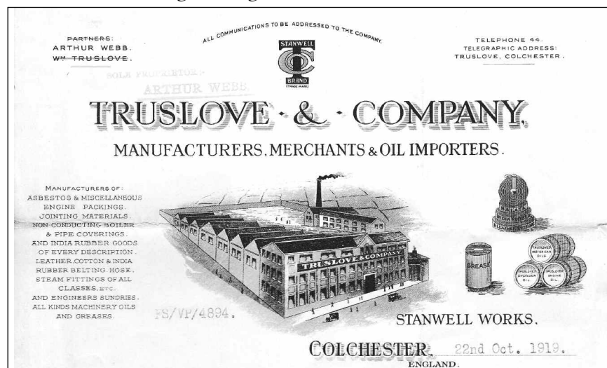
Letterhead of October 1919 with an illustration of Stanwell Works and showing Arthur Webb now as sole Proprietor
