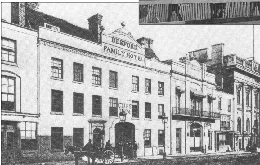
Above: Mr Samuel Besford was at the Cups Hotel from 8th June 1872 until his lease expired at Michaelmas (29th September) 1885, after which the re-building of the hotel commenced.
