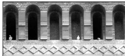
Picture 3 - Detail from 'Jumbo', the water tower.
